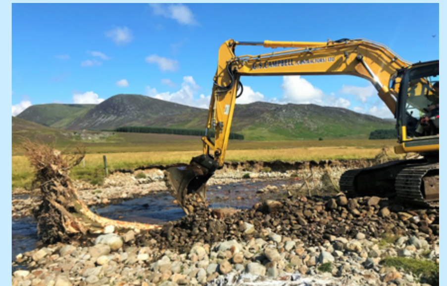
Installing large woody structures on the River Calder. ©Spey Fishery Board
