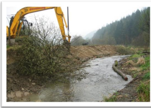
Figure 18. A. Clywedog 2009: Repair in progress
