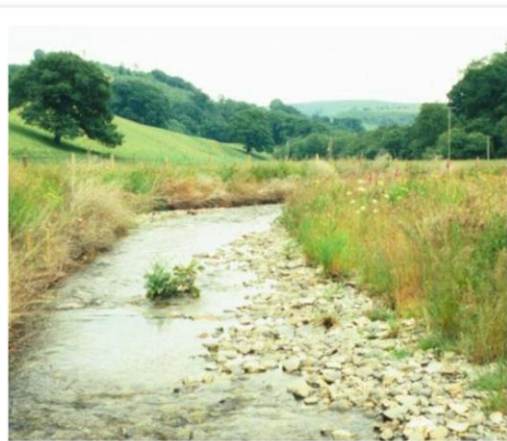
Figure 16. A. Clywedog 1999: 1 year after restoration. Note revetment consisting of Alder logs and tree tops, fence. The stream has started to narrow and many riparian species of plant have returned
