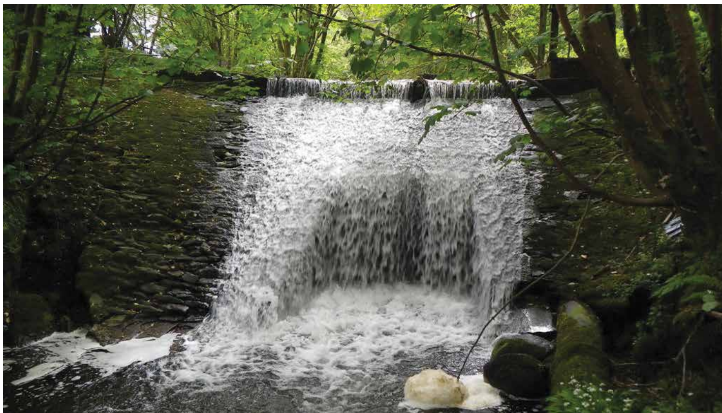
The creamery weir, on an important tributary of the Tarff water in Galloway, cut off about 10km of spawning habitat.
