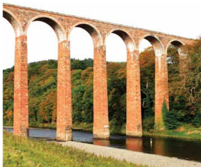
River Tweed at Leaderfoot viaduct.
