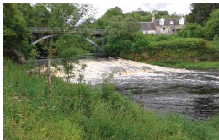
The Millheugh Weir, River Avon, South Lanarkshire.
