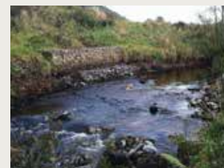
After: Structure removed and with it, the barrier to fish migration
