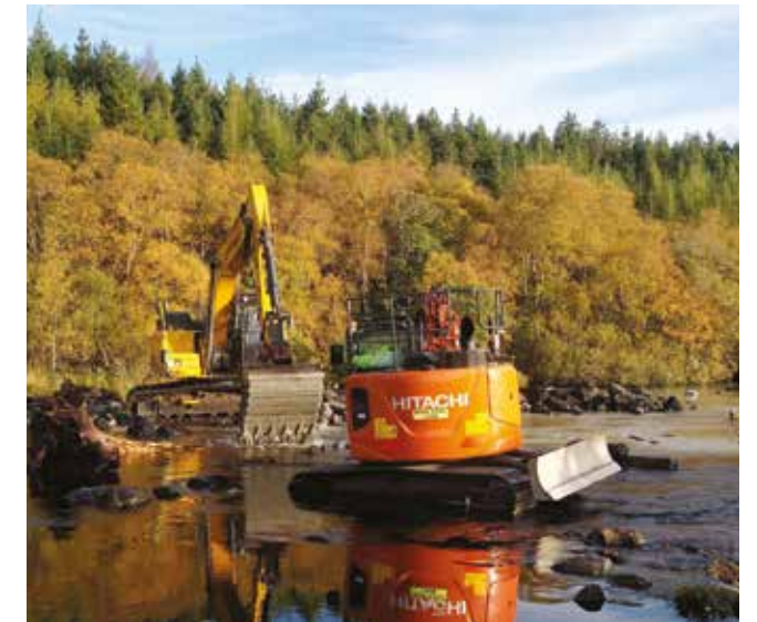
Contractors installing large woody structures.
