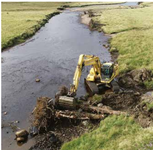
Installing the large woody structures in the headwaters of the River Spey.
