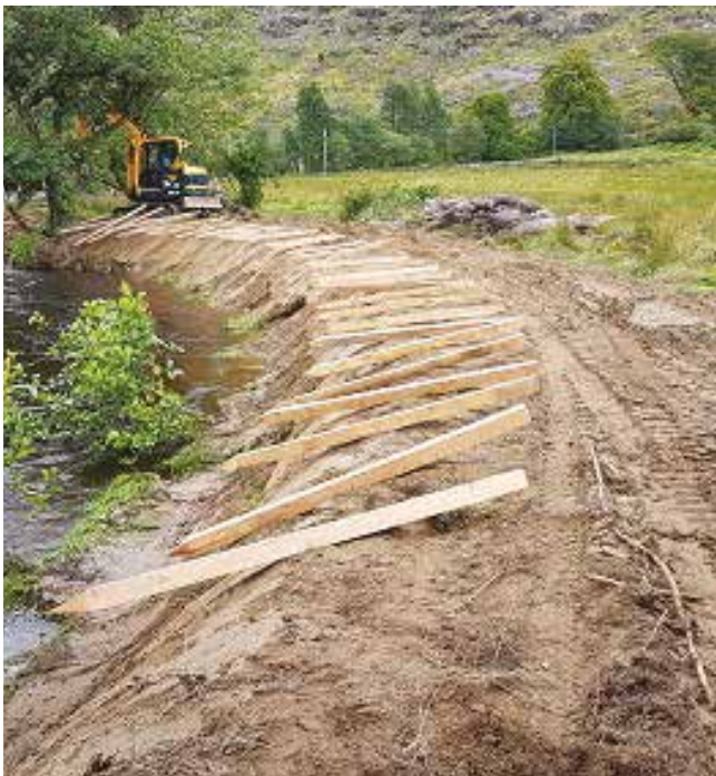
Examples of green bank revetment work on watercourses on the Cowal peninsula - these will help reduce sedimentation
