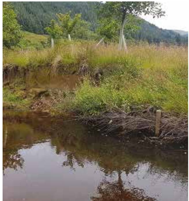
Examples of green bank revetment work on watercourses on the Cowal peninsula - these will help reduce sedimentation
